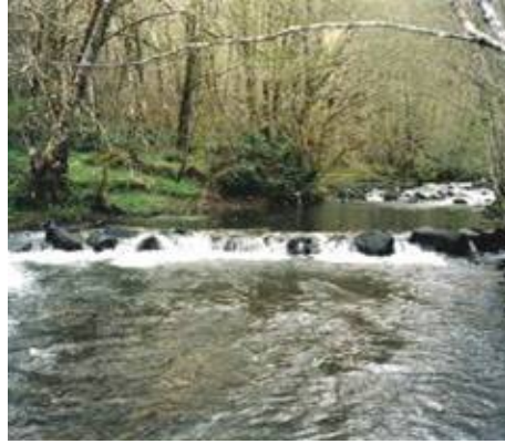
Log weirs placed in a small coastal Washington stream to create pools and habitat for coho salmon. NWFSC.
